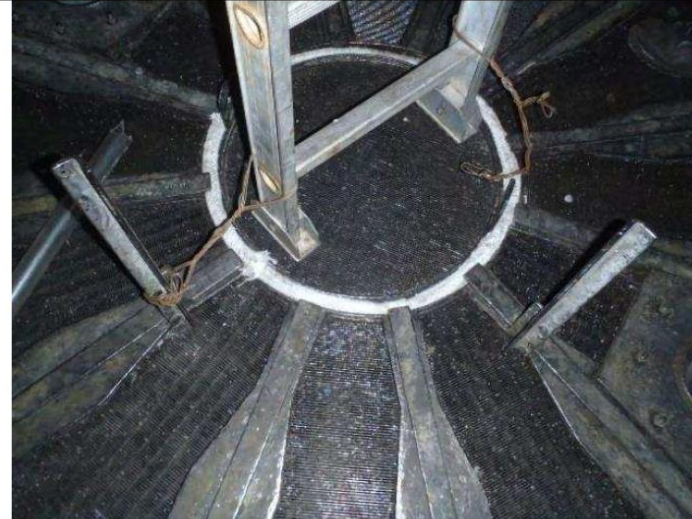
The catalyst support grid center pieces considered sound
